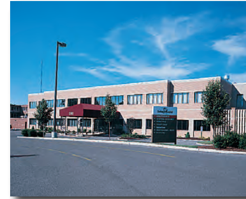
Defiance Hospital Medical Office Building, Defiance, OH
